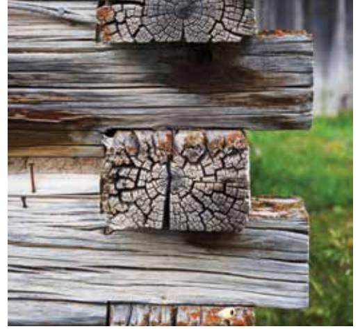
Details of log construction. Photo, Wayne Bingham
